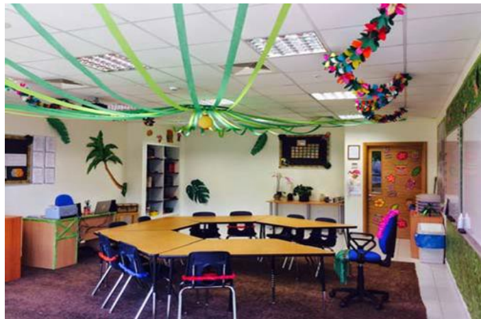
Hanging decorative material will quickly spread a fire across an entire room. Burning debris will drop down onto students. Paper, furnishings and other combustibles will be ignited. Safe exit through classroom doors may be blocked.
