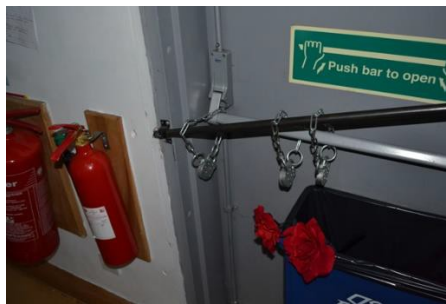
Blocked/chained exit.
